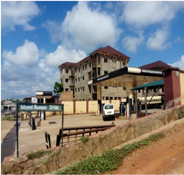
Plate 7: Building Conversion to Hostel beside Filling Station at MFM Junction, Tanke. Source: Author's Field Survey (2019)
