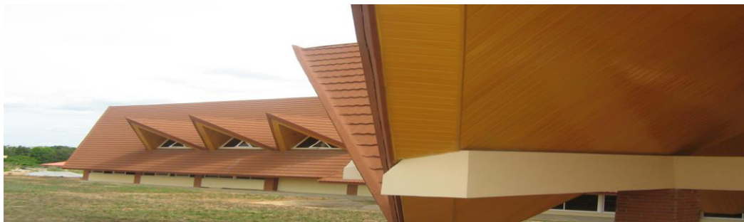
Plate 10 : View of the Roofing sheet
