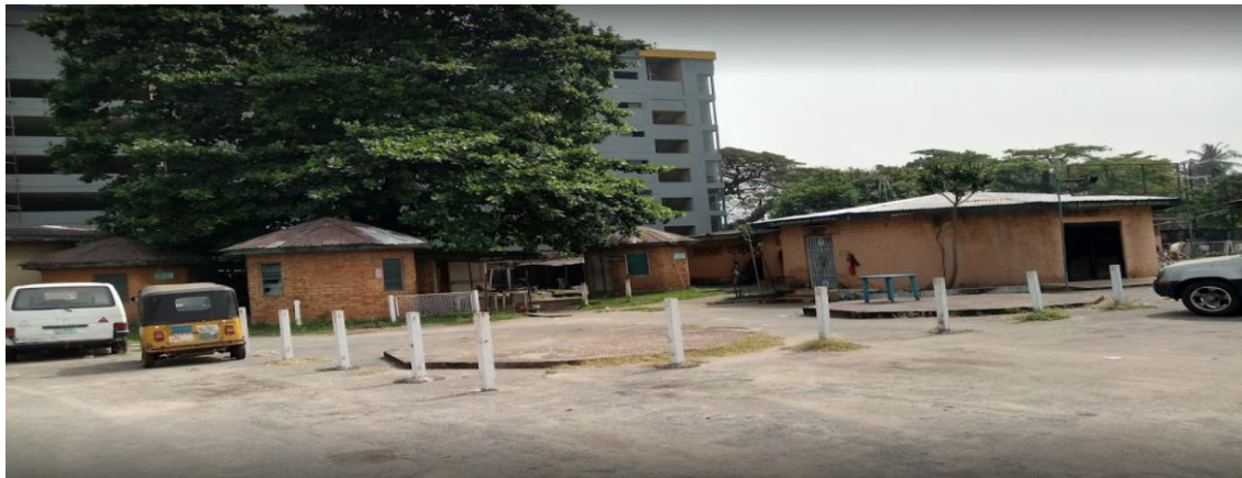
Plate 4 View of the supporting Building facilities; Museum Kitchen and Craft village
